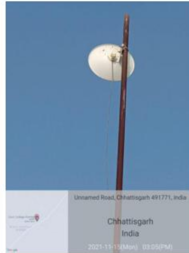
Point to Point Internet Connection in Our College
