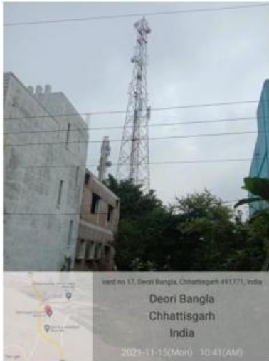
Point to Point Internet Connection BSNL Tower
